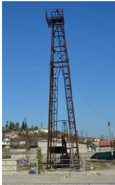
Fig. 10-13. Industrial ruins in Kuçova [photo by the author, 2016]
