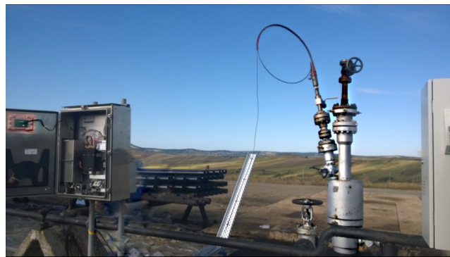
Fig. 4. Wellhead equipment showing fiber optic monitoring integration
